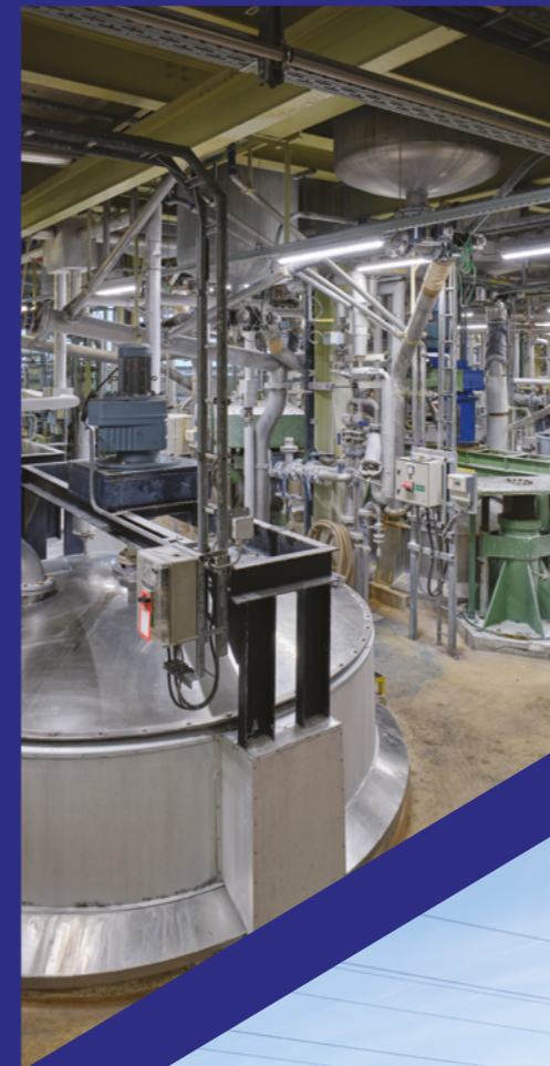
Coating kitchen (Building 929)
