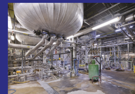
Coating kitchen (Building 929)
