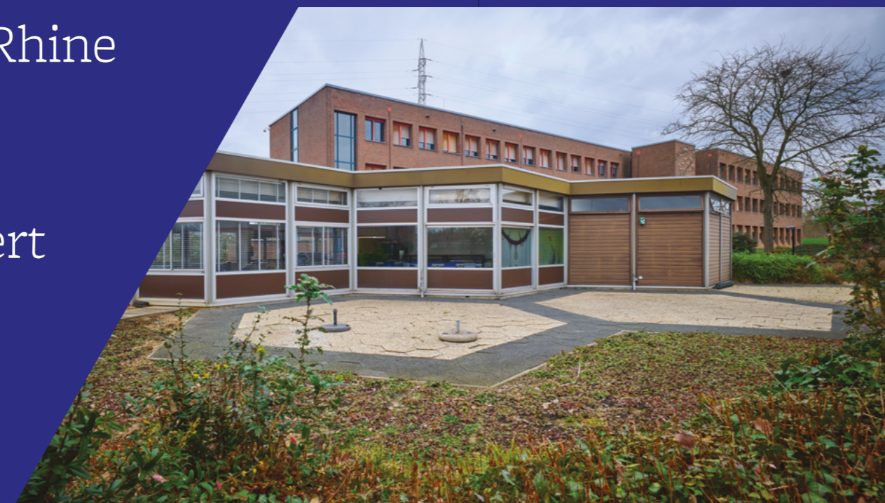
Canteen (Building 949) and Office (Building 980)
