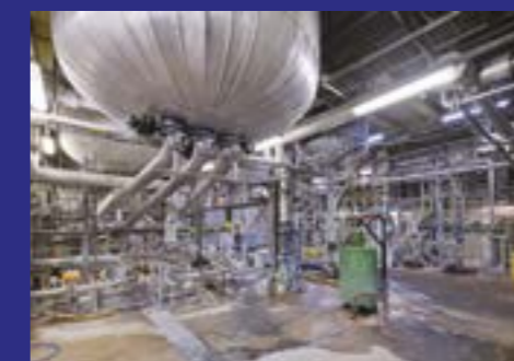
Coating kitchen (Building 929)
