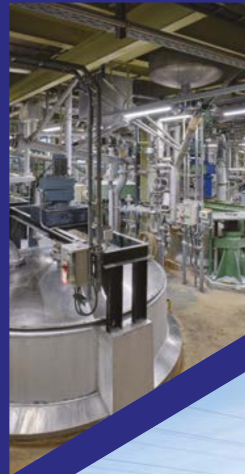
Coating kitchen (Building 929)
