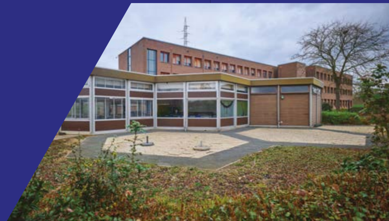
Canteen (Building 949) and Office (Building 980)
